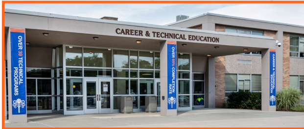
Career and Technical Education at the Amy Bull Crist Area Education Center 53 Gibson Road, Goshen, NY 10924
